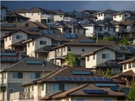
Solar panels on rooftops in Hawaii. Image via NYTimes.
